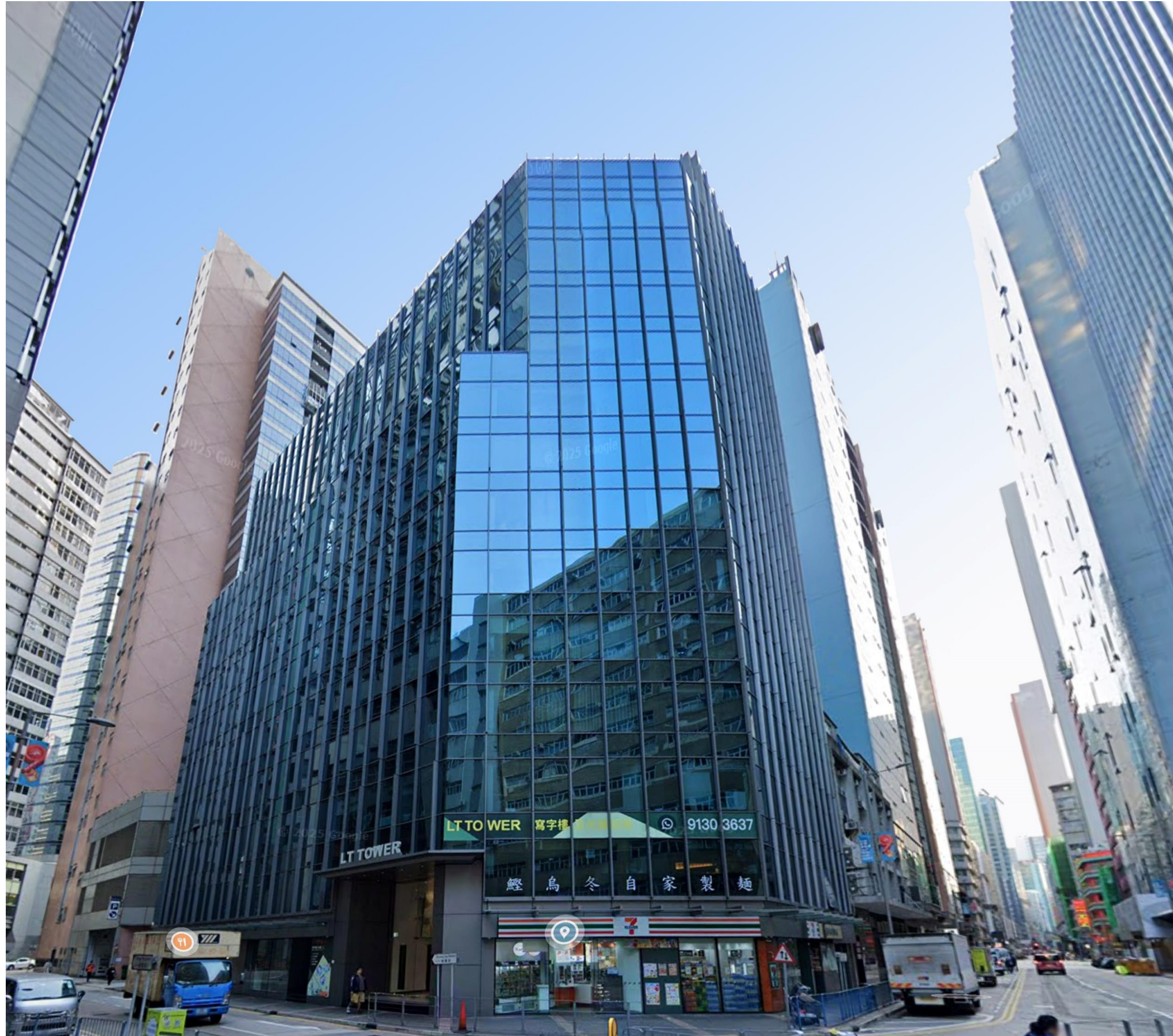
Photo 1 - Western facade of the building
